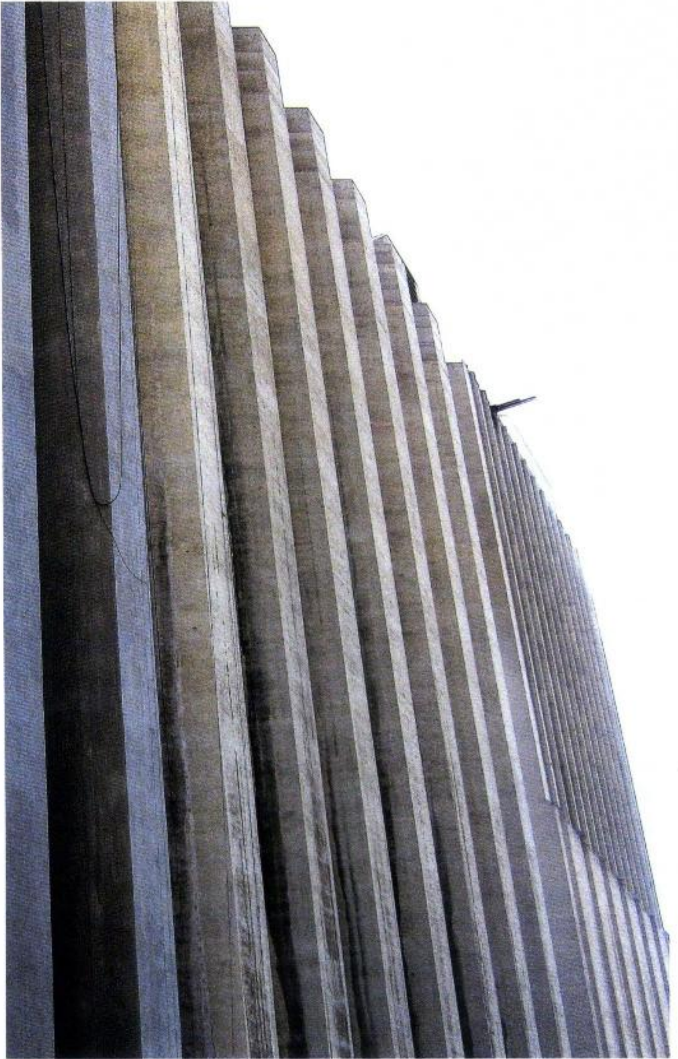
Maize silos repaired with a.b.e. Construction Chemicals products
